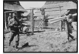
Barackenbau in Tucholka.
