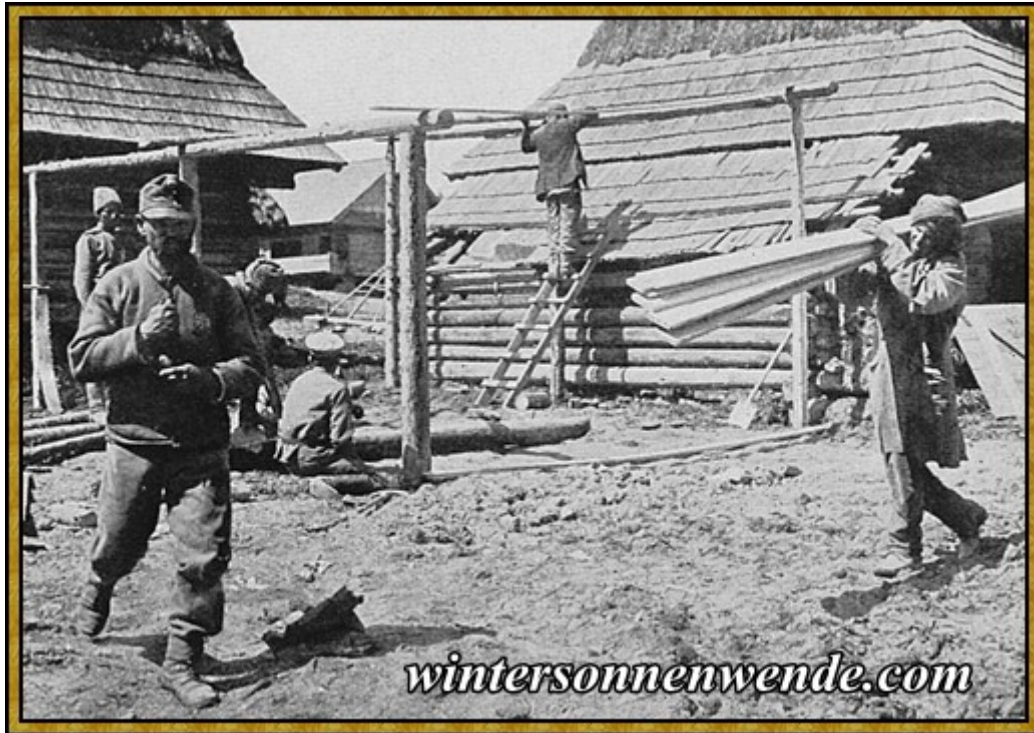
Barackenbau in Tucholka.
